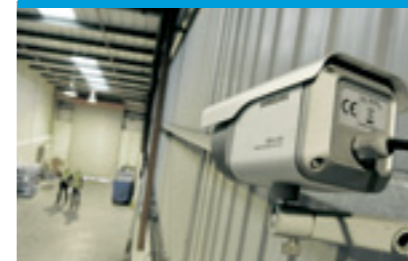
The SIR-4150 features extensively throughout this installation, both internally and externally, providing effective 24-hour surveillance thanks to the units integrated IR LEDs
