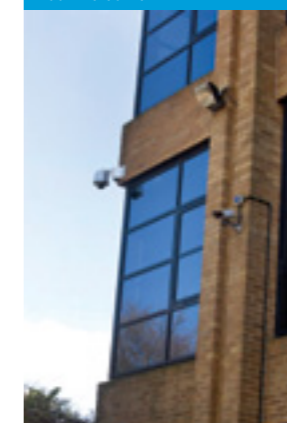
A mix of Samsung Techwin speed domes and static cameras protect the building's exterior.
