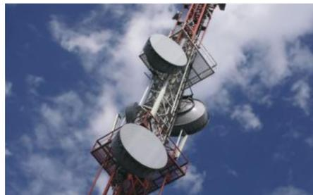
Base station, fixed and mobile telephone Network and radio link system
